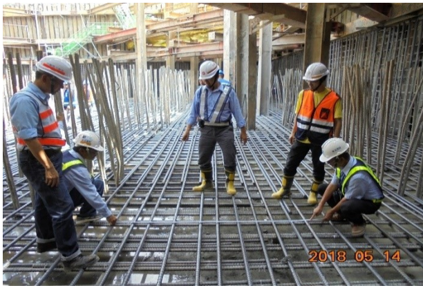
Fig. 6. The inspection of foundation by the authors.
