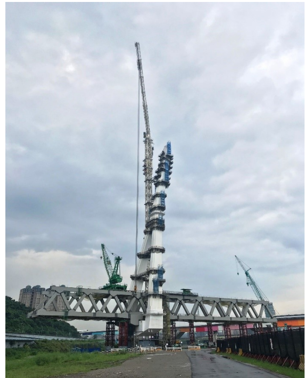
Fig. 10. The site photo of the erection system for truss frame (ESTF).
