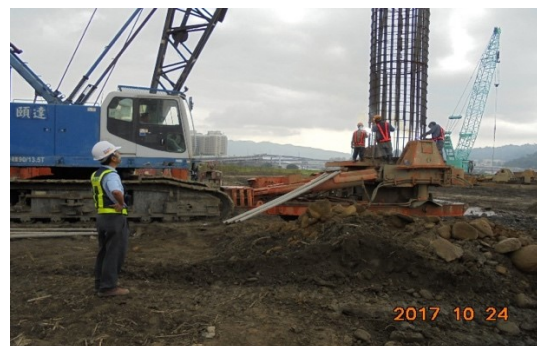
Fig. 5. The construction of the 2m-diameter piles supervised by the first author.
