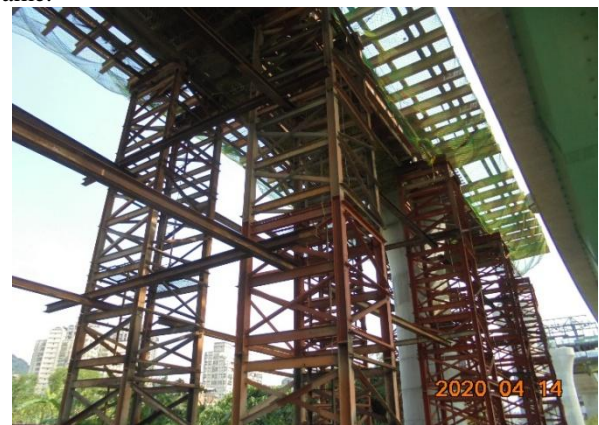
Figure 7: The typical site installation of the steel truss frame
