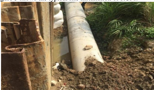
Figure 5: The typical site installation of RCPs
