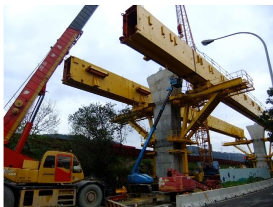
Figure 9: The typical site assembly of the advancing shoring system
